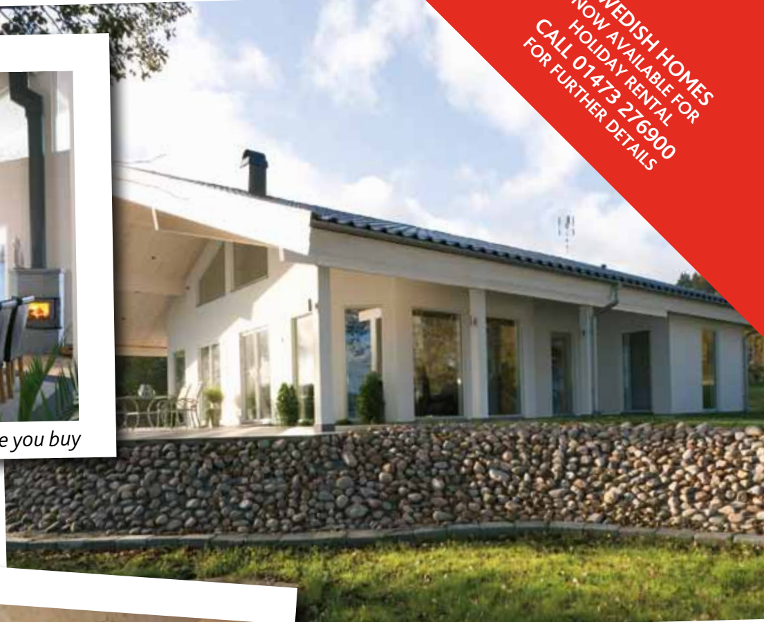
Climate resistant • Reduced on-site build time
