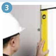
3. Ensure frame is square and plumb
