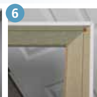
6. Fit and fix architraves in place
