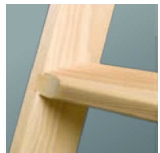
Treads with non-slip grooves
